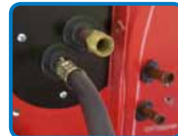
A/C and Heater Fittings Pass Through Existing Factory Holes In Firewall.
